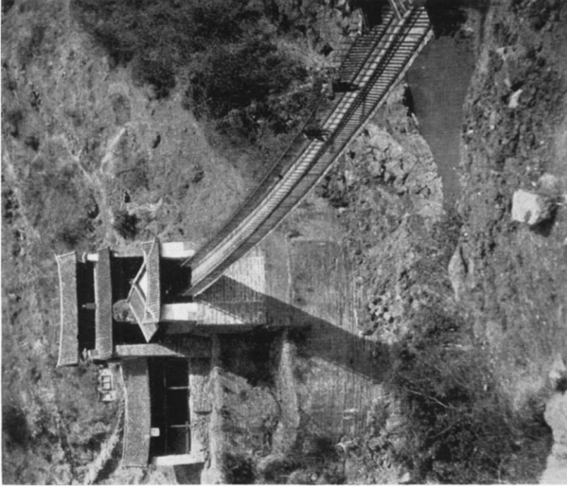
5. CHAIN BRIDGE OVER THE MEKONG
